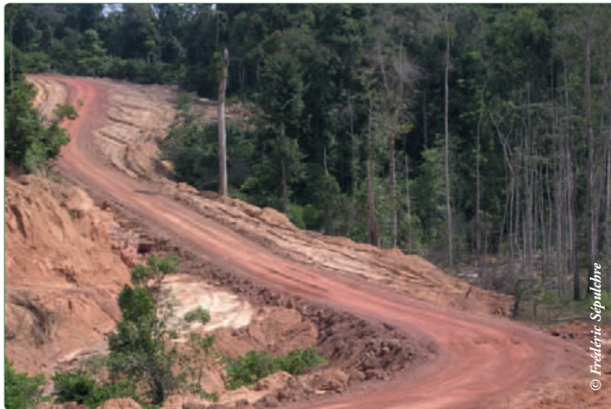
Photo 10.8: Signs of erosion and obstruction of valley floor from the construction of a forest road, Gabon
