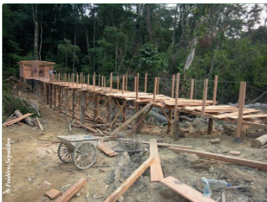
Photo 2.10: Construction of latrines for workers' camp, Gabon
