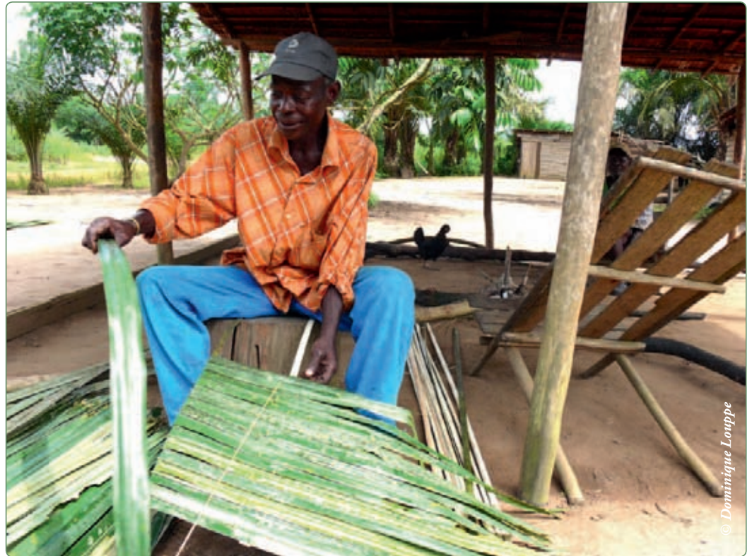
Photo 10.13: Fabricating roofing from palm leaves – Congo
