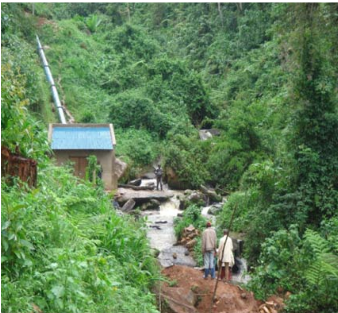
Figure 5. Hydro-electric station (37 kw) serving TCCB, radio station, and village of Kasugha
